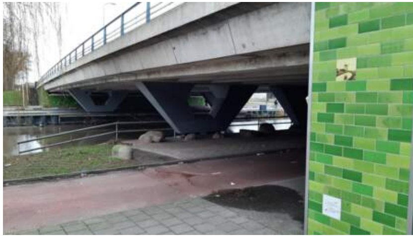
Side view of the bridge and drawings with indications of GPR data collection
