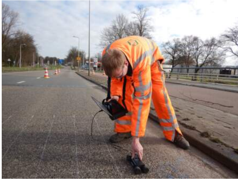
Using the Profometer on the bridge
