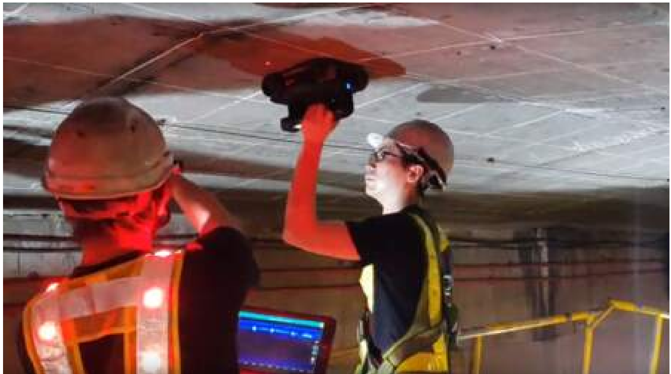
The Proceq GP8000 GPR scanning thick concrete
