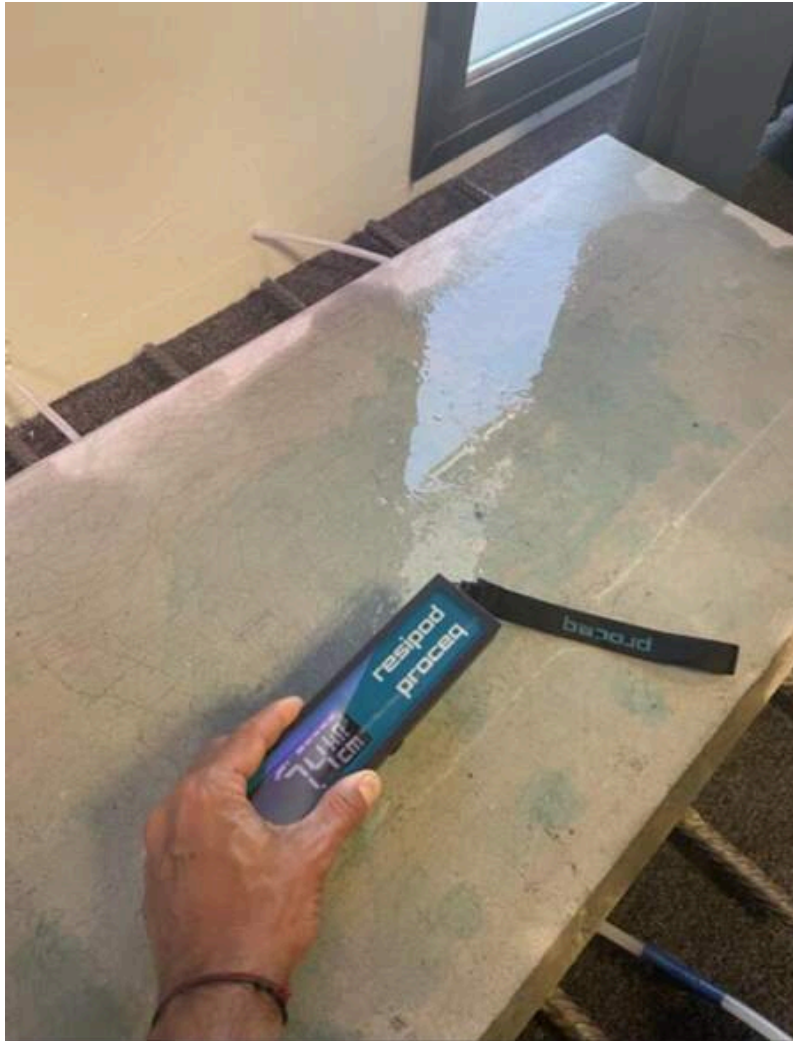
Concrete resistivity results using Resipod
