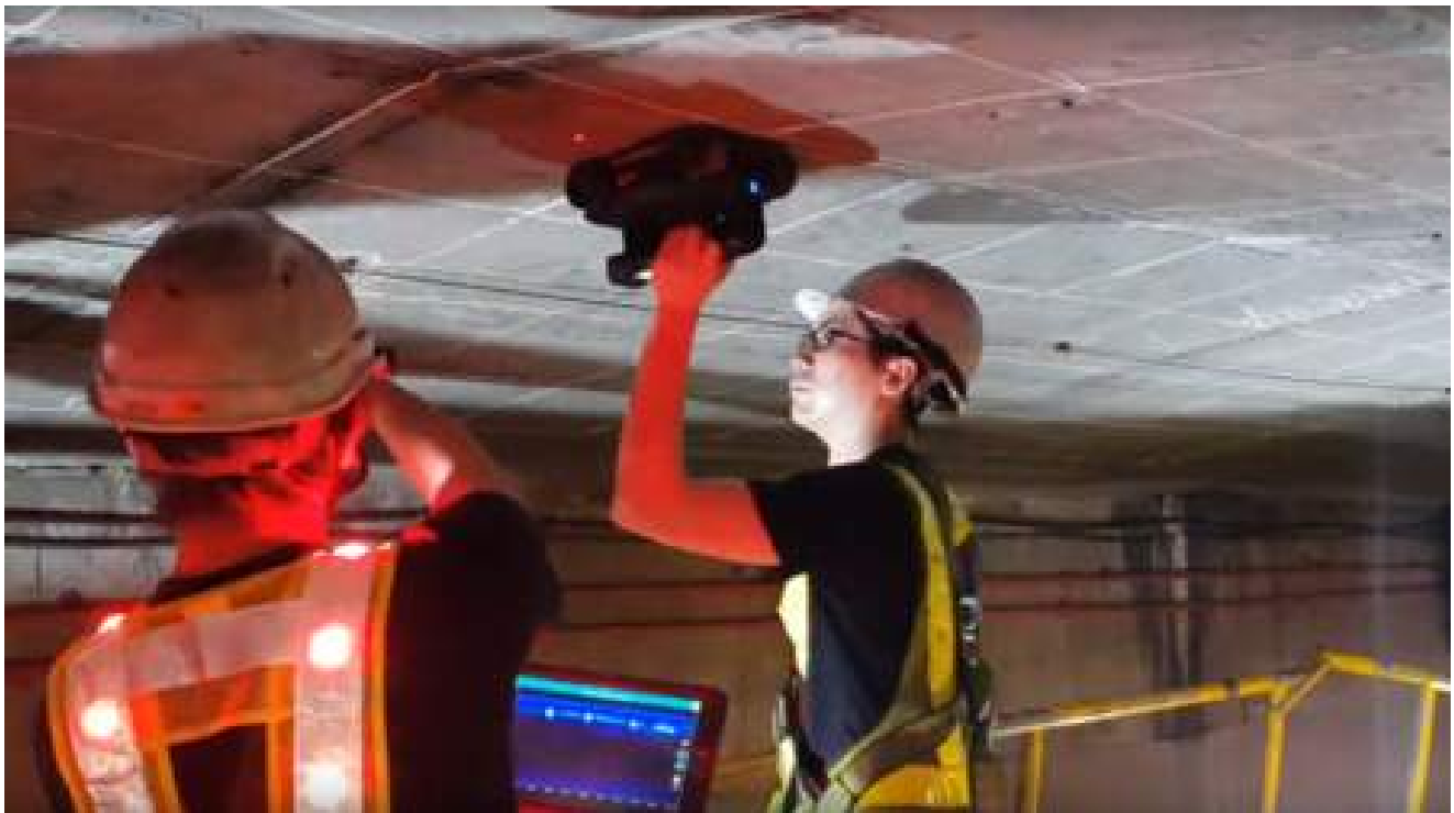
The Proceq GP8000 GPR scanning thick concrete
