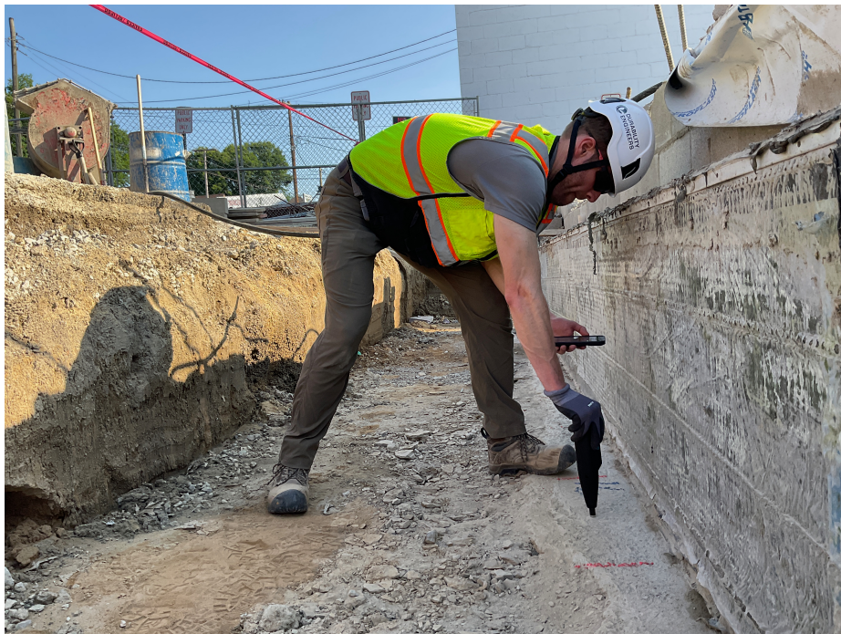
Durability Engineers onsite using the Silver Schmidt Hammer
