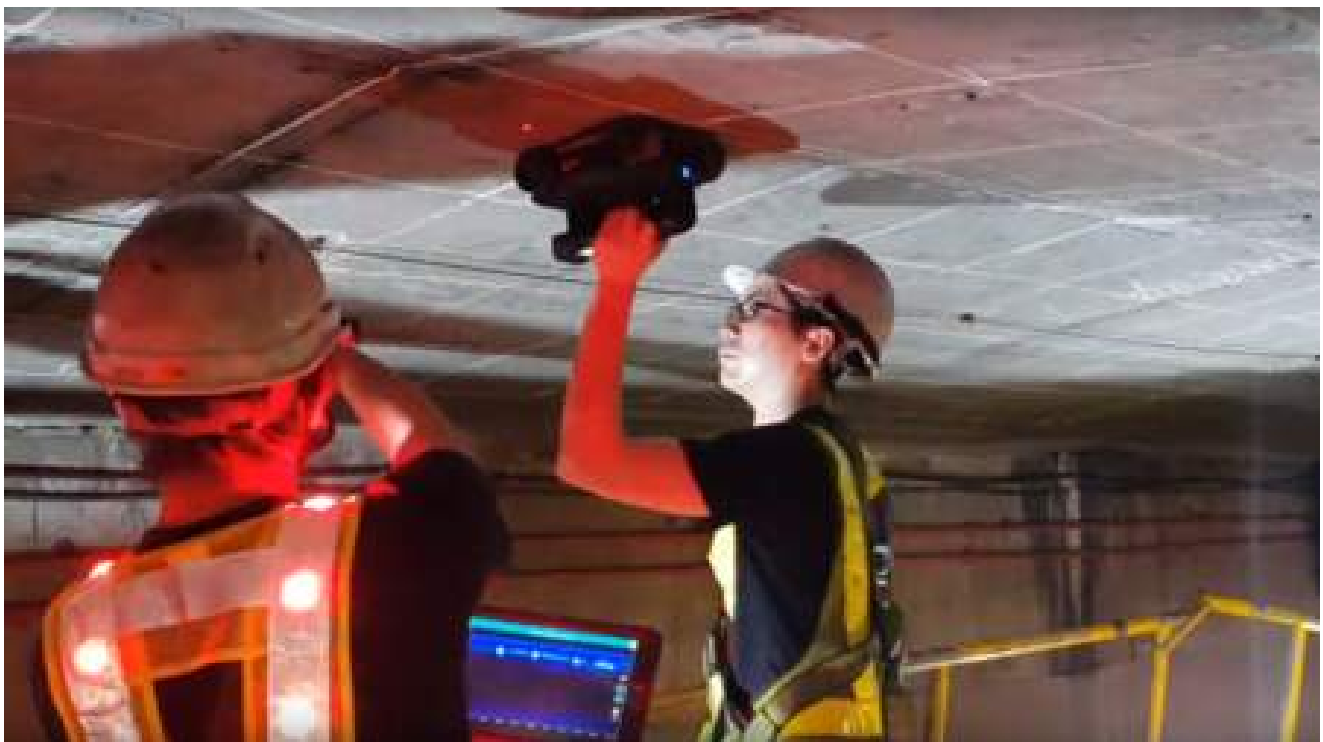
The Proceq GP8000 GPR scanning thick concrete
